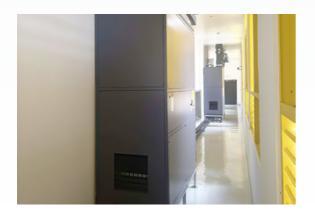
In 2024, Hoyinn collaborated with customers to research anti-freezing technology for the spray system of indirect evaporative cooling units. By adding technical means such as electric valves on the inlet pipes, submersible pumps, temperature sensors, and water tank agitation pipes, the system reduces the repeated draining and refilling of the spray water pool during large diurnal temperature variations. The campus can save approximately 41,000 tons of water annually.
