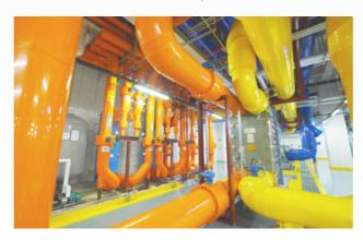
In 2024, to reduce the energy consumption of diesel generator in winter, ND18 adopted plate heat exchangers to recover waste heat from the liquid cooling system and utilize it in the cylinder jacket cooling system of diesel generators, thereby improving winter start-up performance. For two diesel generator buildings, a total of 4,100 GJ of heat can be recovered annually, saving 1.1 million kWh of electricity and reducing carbon dioxide emissions by **745** tons.
